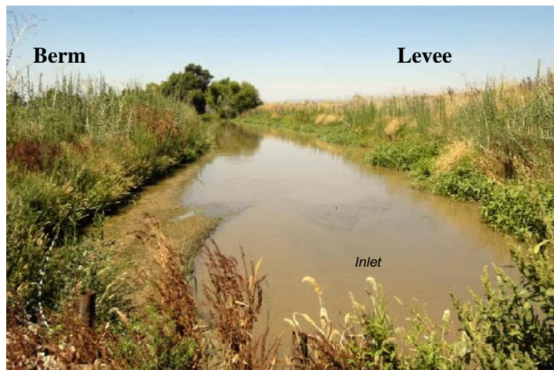
Figure 3. Inlet of wetland
