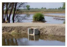
• Minimize local flow velocities around the water control structures to reduce erosion and re-suspension of sediments
