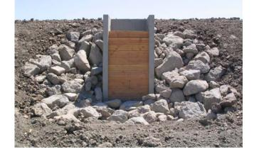
wetland cell is draining and localized flow velocities are relatively high. If velocities are expected to be relatively high, rip rap should be installed for protection.
