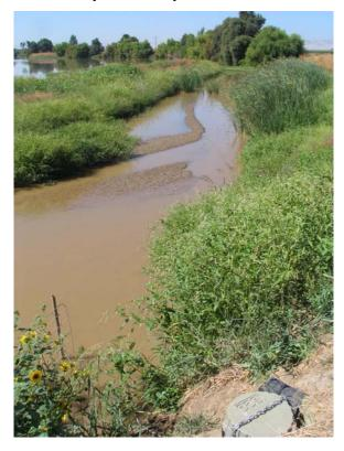
The basins should be sized to facilitate the settling of the majority of sediments. This is dependent on the incoming flow rates and the amount/type of sediments entering the wetland - the finer the materials, the longer it will take for the material to settle out.
